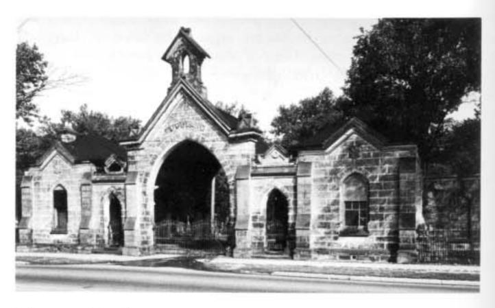
The Woodland Cemetery Gatehouse (above), in a state of imminent collapse, was disassembled in 1996. The work was carefully documented with each stone marked and stored, to await reconstruction when funding is available.
